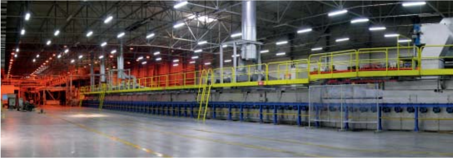
Impressive dimensions: The total length of the float glass facility is several hundred metres.
