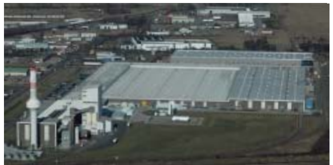
Euroglas float glass factory Haldensleben, Germany
